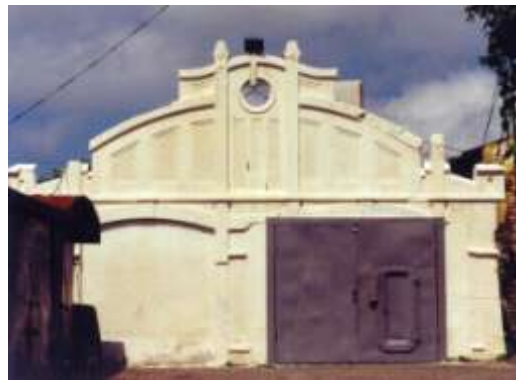
Poti. Carriage parking. Architect unknown. Beginning of the 20c. Tbilisi.
